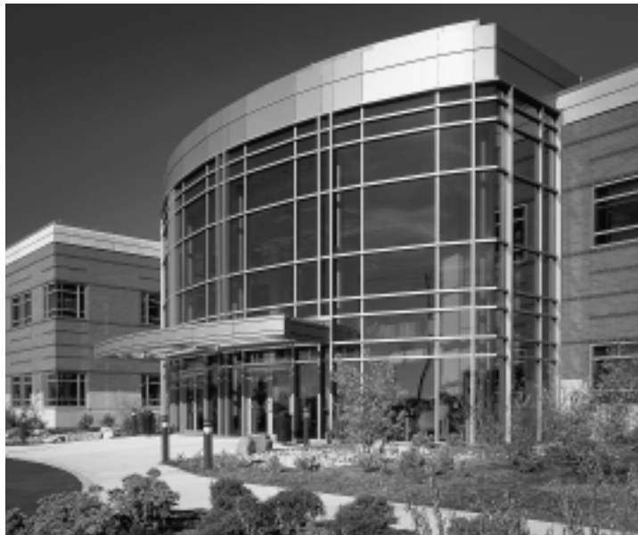
Philips CSI's office facility, Greenfield Corporate Center, Lancaster, Pa.
